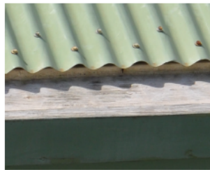
View of Staggered Metal Panel Fasteners at Eave.
