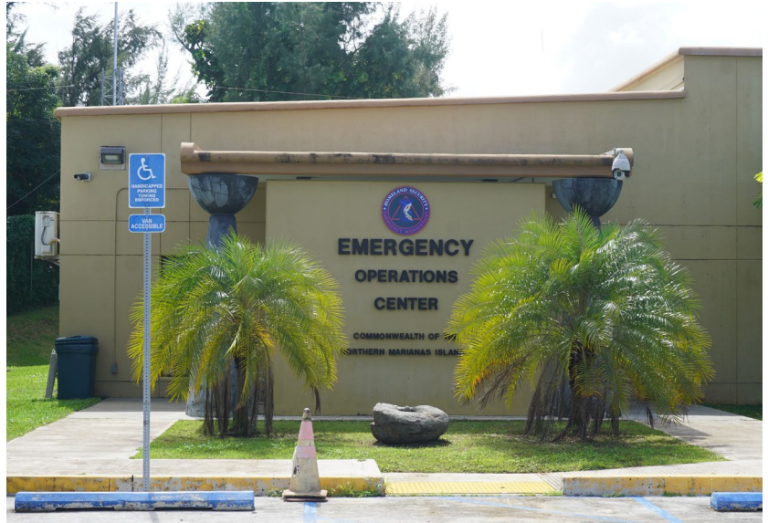
Figure 2. Entrance to CNMI Emergency Operations Center.
