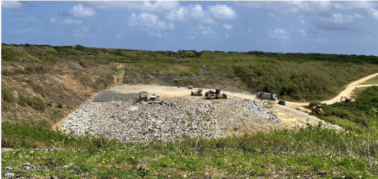
Figure 37 Marpi Landfill Cell 2
