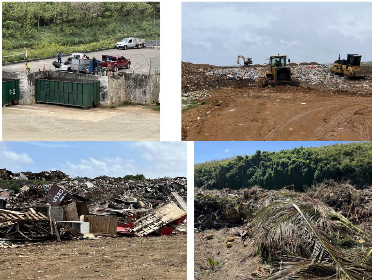
Figure 12 Marpi Landfill and Wood Waste Areas
