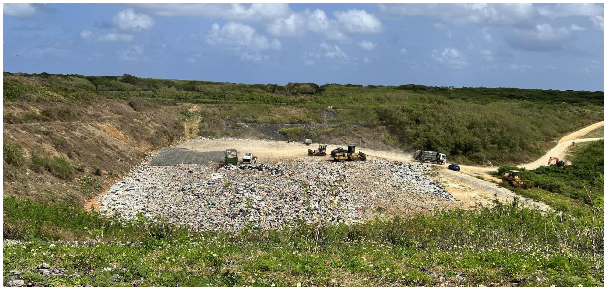
Figure 36 Marpi Landfill Cell 2
