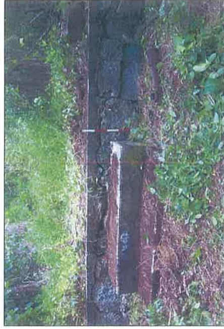
Figure 21. PL-12, Concrete Slab with Stairs (note cut blocks in construction)
