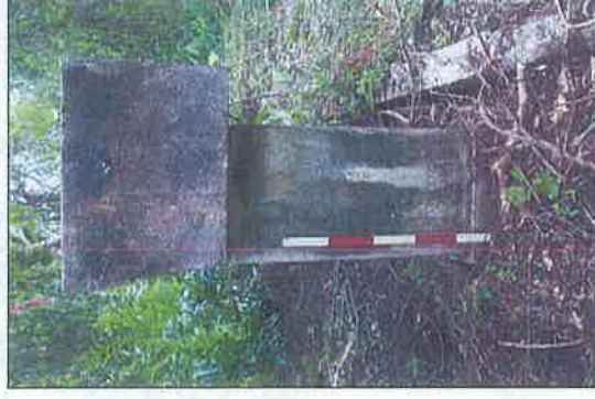
Figure 9. PL-4: Detail of Concrete Trough (view to N)
