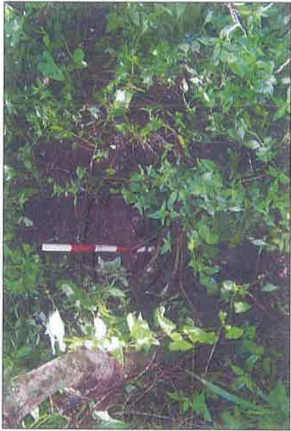
Figure 12. PL-5: Metal Culvert (view to E)
