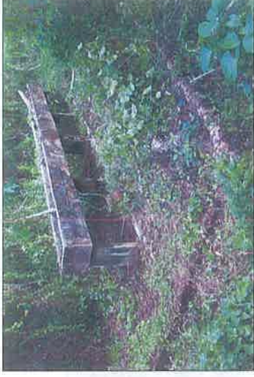
Figure 8. PL-4: Pedestaled Concrete Trough (view to NW)
