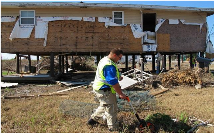
Category A: Debris Removal from Private Property (5 of 7)
