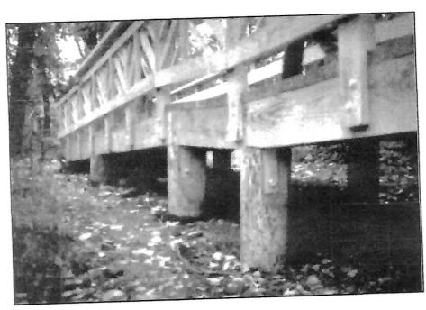
Basically, a boardwalk is a series of connected bridges, each with a span as long as is practical, perhaps 8 to 40 feet. At most wetland sites, longer stringers are not practical because they are difficult to transport. Also, building adequate foundations for the long spans often requires large pieces of specialized equipment that cannot negotiate unstable soil.
