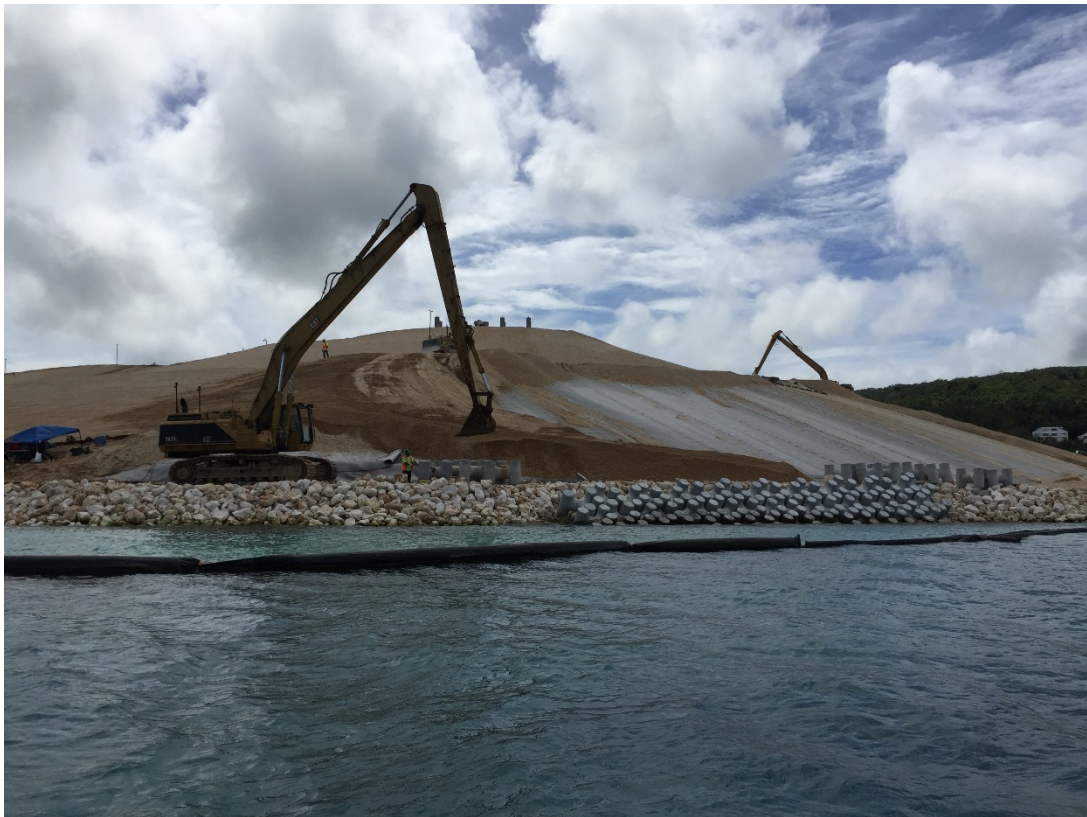
Figure 14 Revetment construction on the Puerto Rico Dump Site
