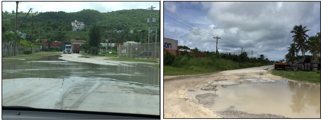
Figure 17 Local Port Roads highlighting poor drainage and condition, 2016
