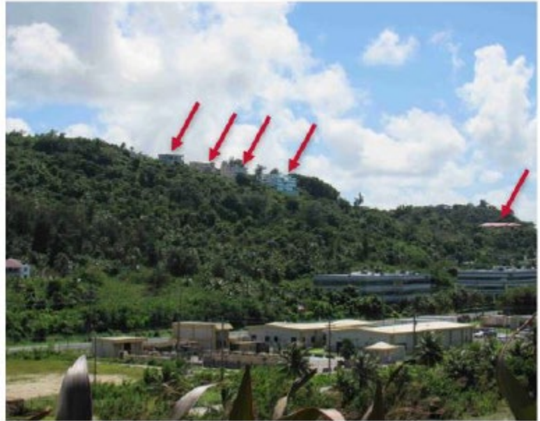
Figure 4.2-4. Homes located on a ridgeline, like these in Saipan (indicated by red arrows), typically experience higher wind speeds than homes on lower, flat terrain.
