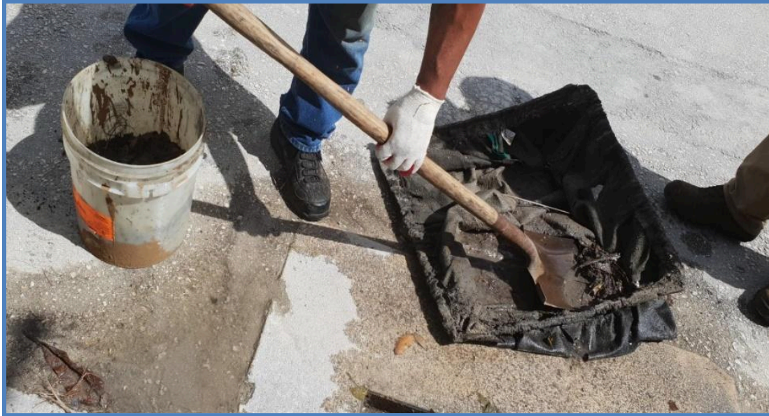
Figure 4. Storm Drain Guard Maintenance
