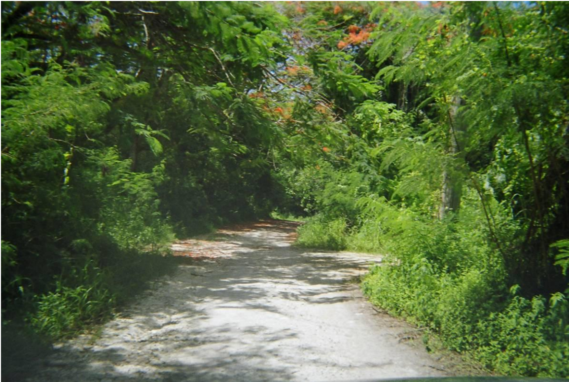
Figure 64: Existing Lau Lau Bay Drive
