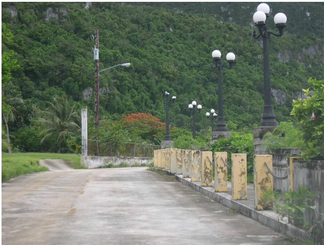
Figure 80: Existing Bridge with limited travel-way width on Route 100
