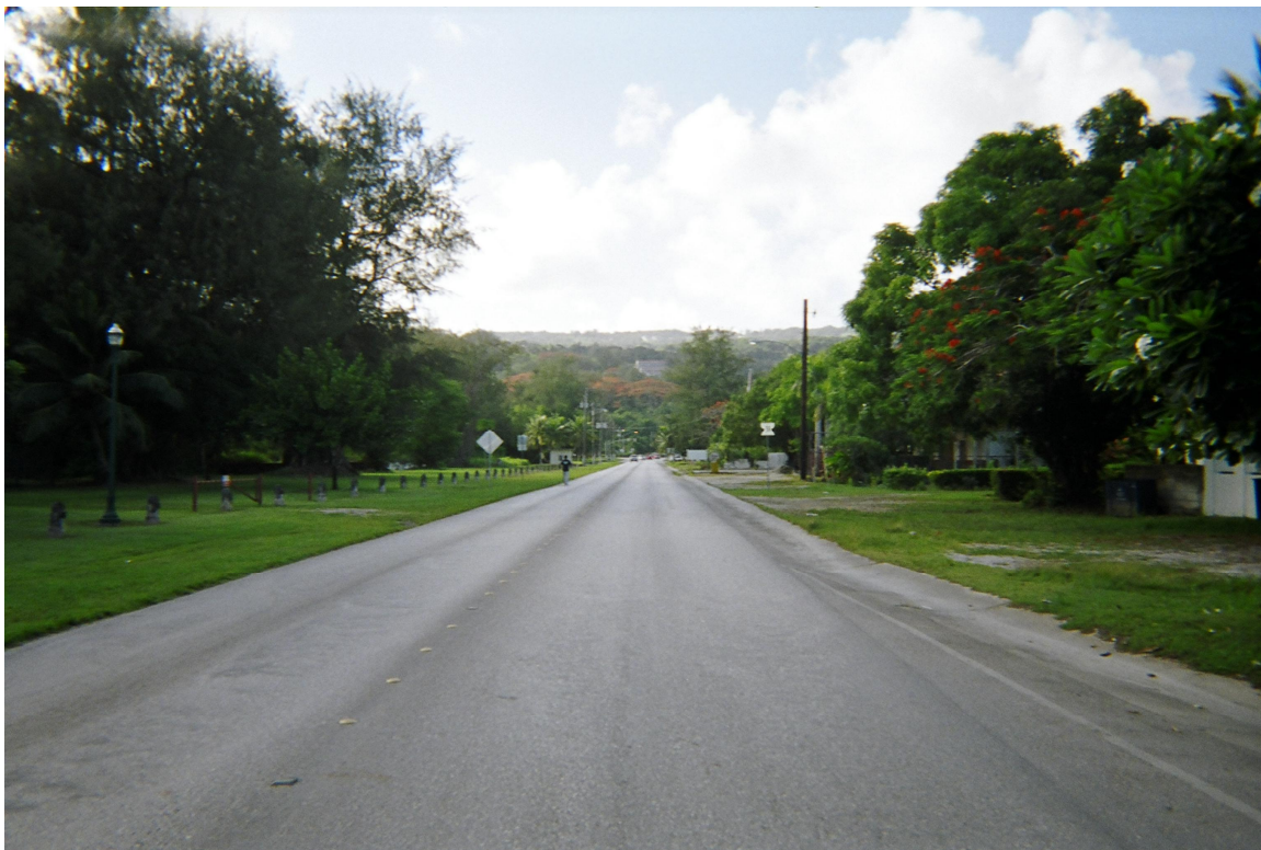
Figure 68: Existing Micro Beach Road
