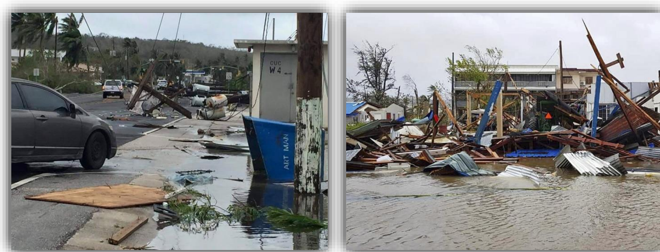
Figure 1.2 Storm-damage to the power distribution system from Super Typhoon Soudelor (left) and wreckage from Super Typhoon Yutu (right).
