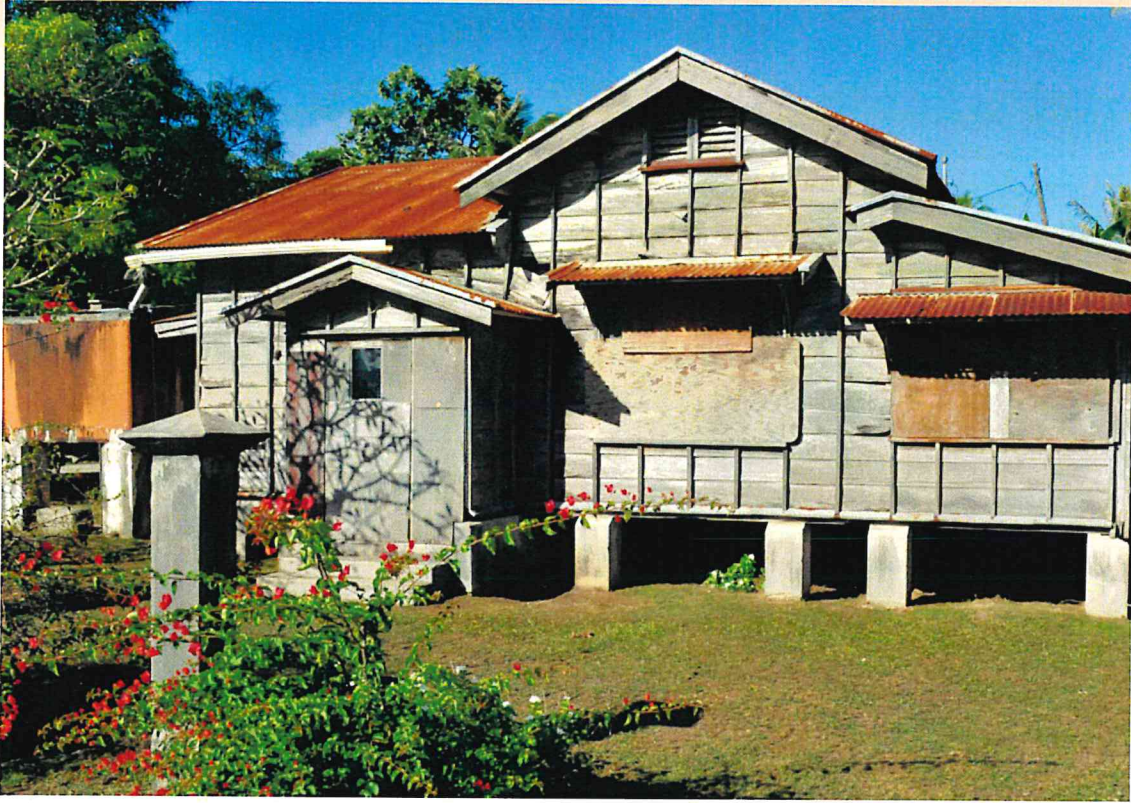
A Japanese era residence in Chalan Kanoa Village, Saipan.
