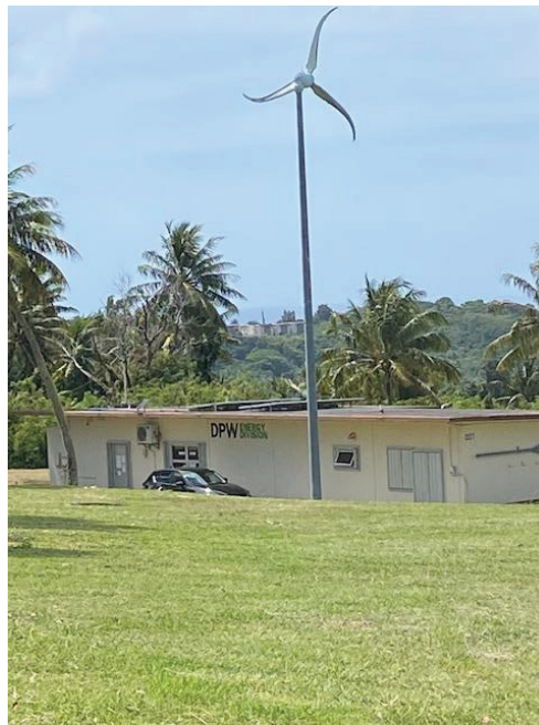
Figure 12. Skystream 2.4kW residential wind turbine demonstration system at DPW Energy Division office.
