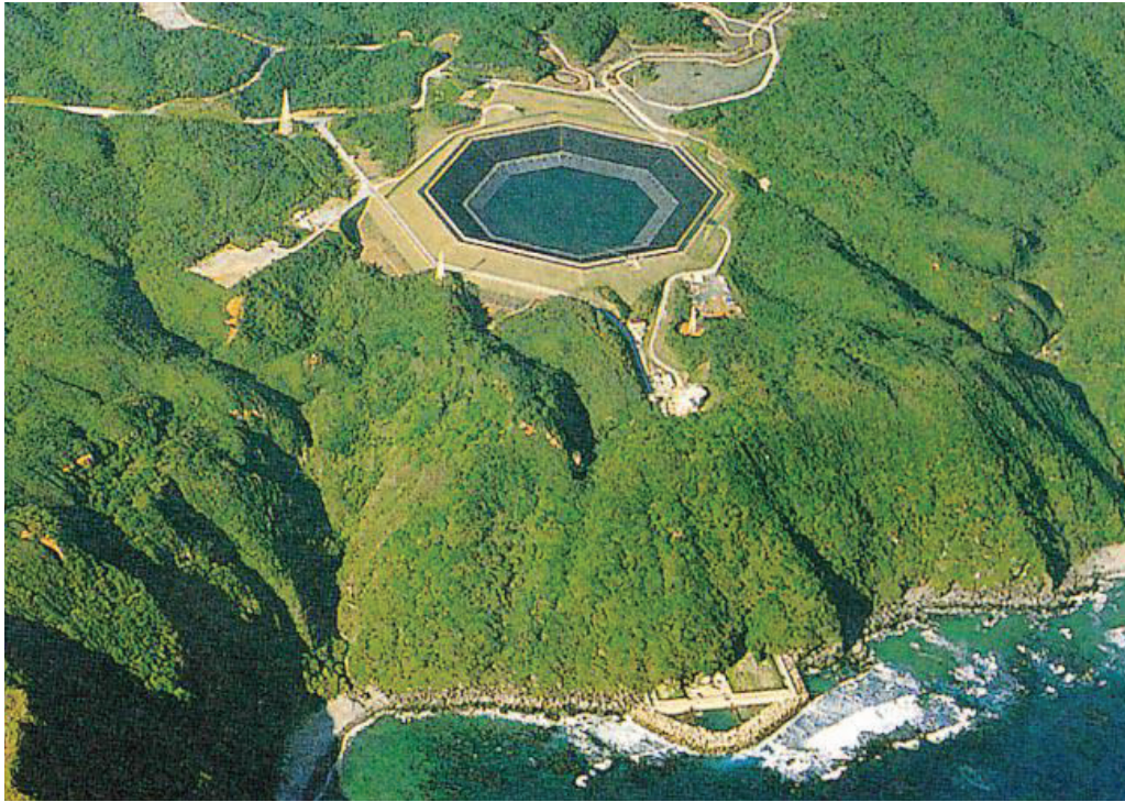
Figure 17 Okinawa Seawater PHES (31.4MW)
