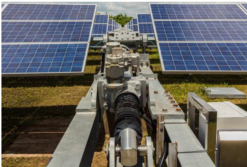
Figure 10. Example of a Ground Mounted SAT System
