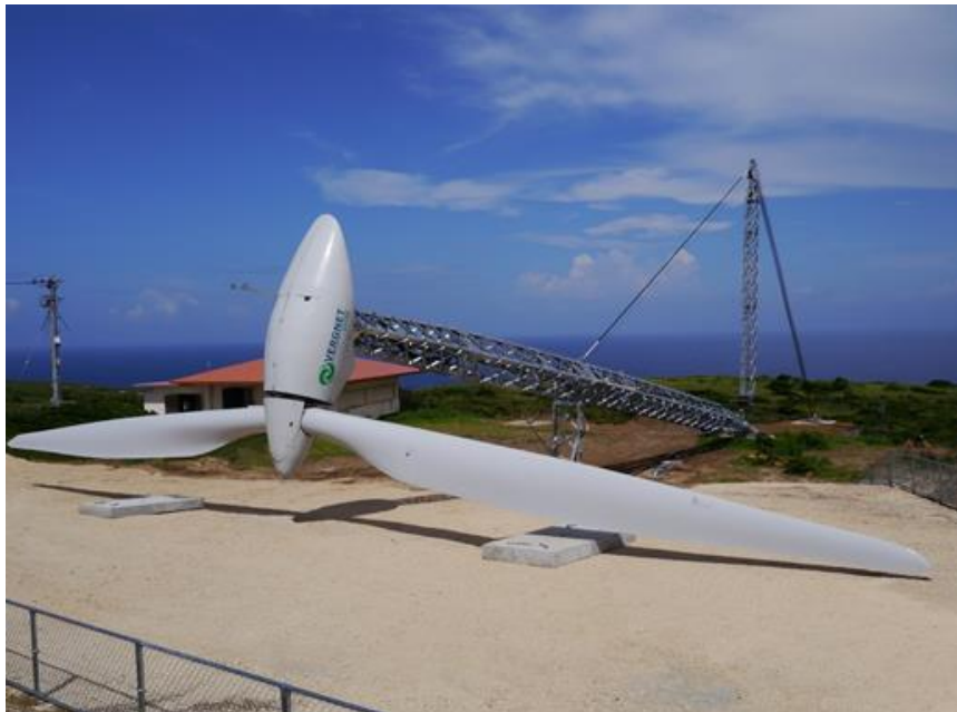
Figure 14. Tilt down Wind Turbine for Protection Against Extreme Wind Speeds
