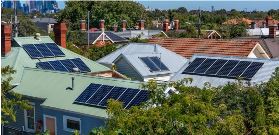
Figure 9. Solar PV Modules Installed on Residential Rooftops
