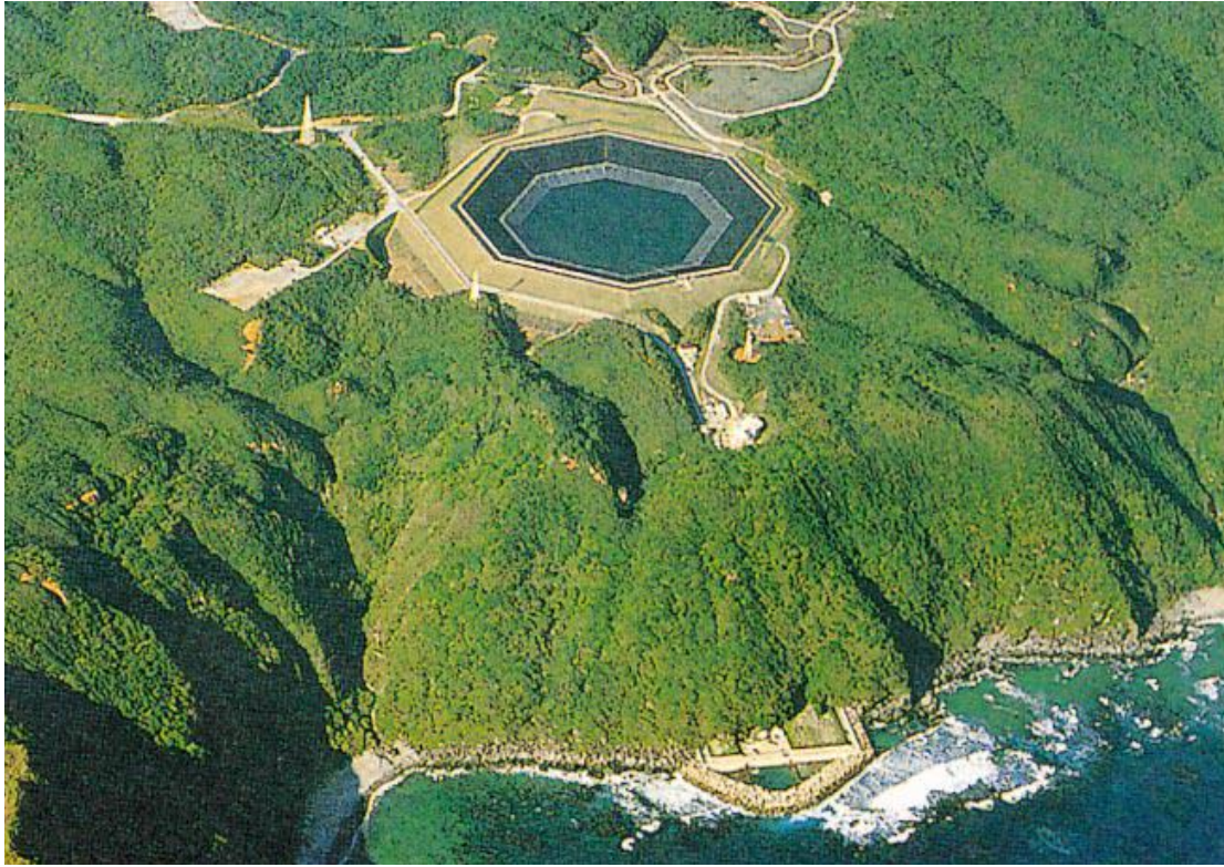
Figure 17 Okinawa Seawater PHEs (31.4MW)
