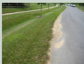
Filter Strips and Buffers
