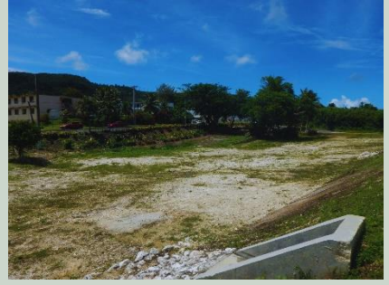
This basin collects runoff between Middle Road and the Federal Court House. Photo Credit: Ross Arriola
