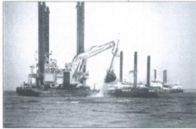
Floating excavators prepare an underwater trench for the Nord Stream 2 pipeline close to Lubmin, Germany on May 15, 2018. REUTERS
