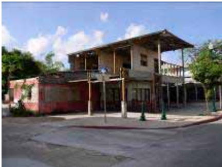
Figure 12. Derelict buildings in prominent tourist-oriented areas detract from Garapan’s identity.
