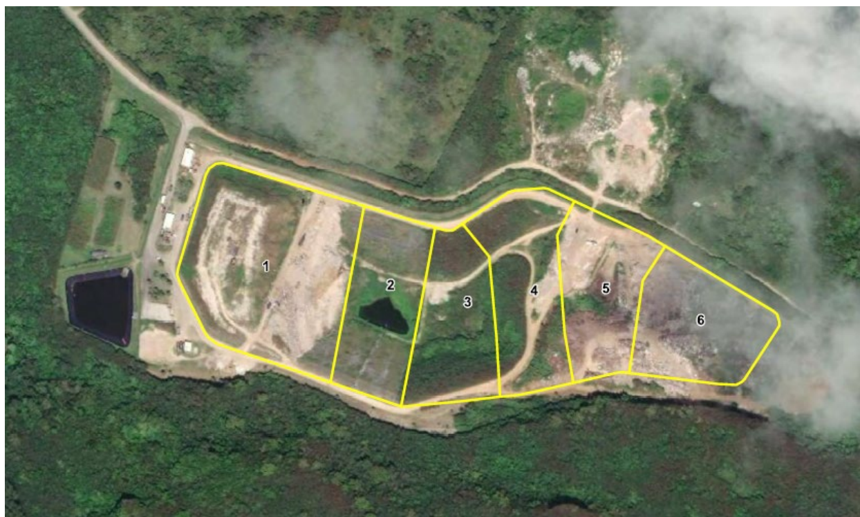
Figure 1. Marpi Landfill cell layout; all structures are west of Cell 1.
