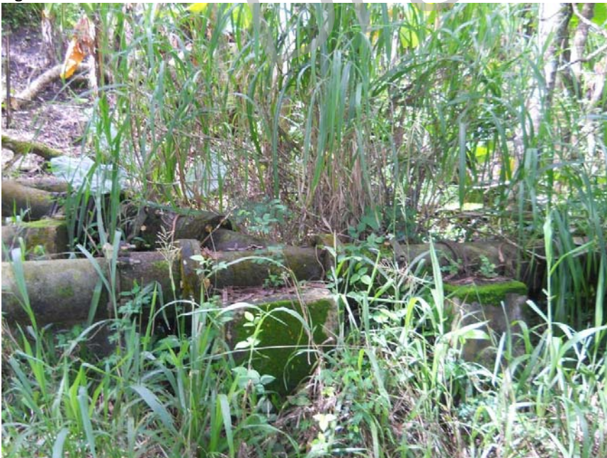
Figure 2.2.2-10. Transmission Line Intersection of the Main and Onan Caves
