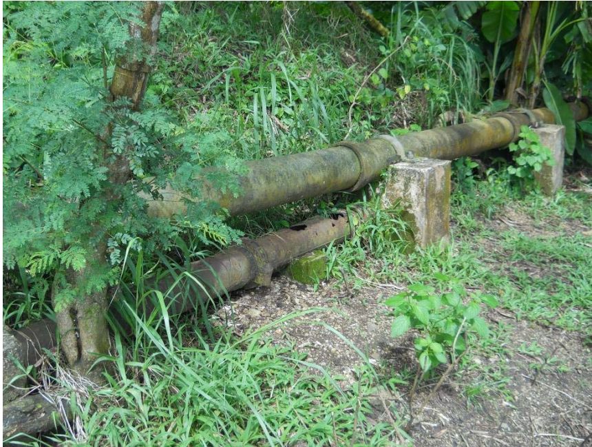
Figure 2.2.2-11. Abandoned Transmission Line Shown Below New 10-Inch Line
