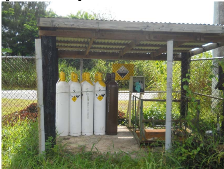
Figure 2.2.2-8. Ginanlangan Tank Site
