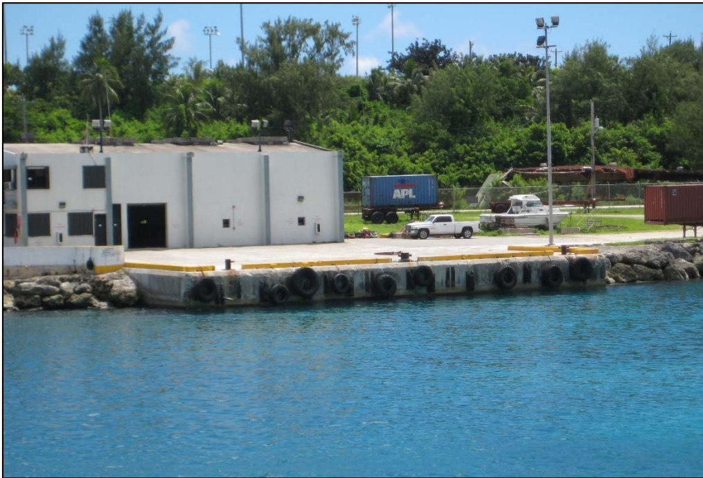
Photo 2. Berth 2 or the “New Dock” with the Port Operations Building is seen from the offshore island looking southeast.
