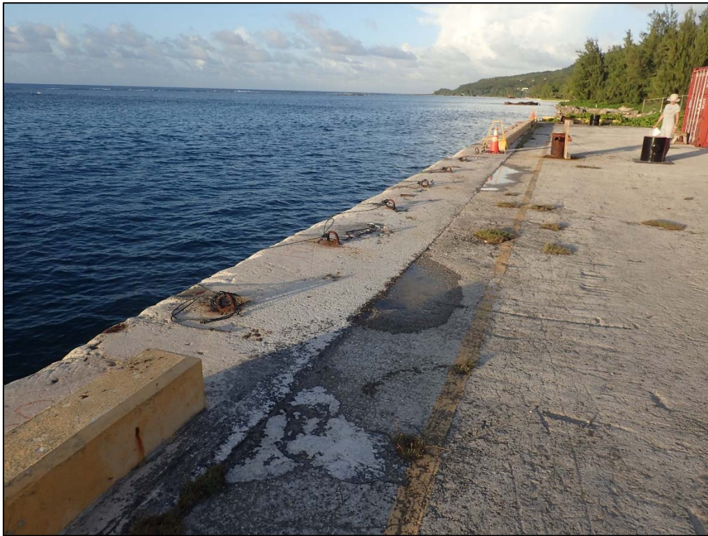
Photo 32. A section of curb was removed at Berth 1 from Station 0+33 to 0+75.
