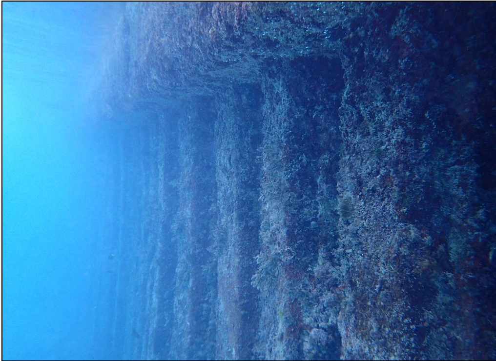
Photo 3. Berth 2 front face sheet pile elevation below water. The pile cap can be seen at the top of the sheet piles.
