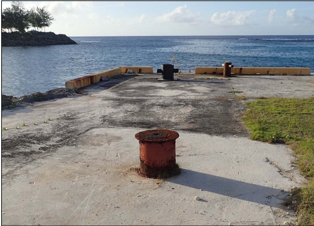
Photo 22. An 18-in. diameter bollard approximately 50-ft behind the face of Berth 1.
