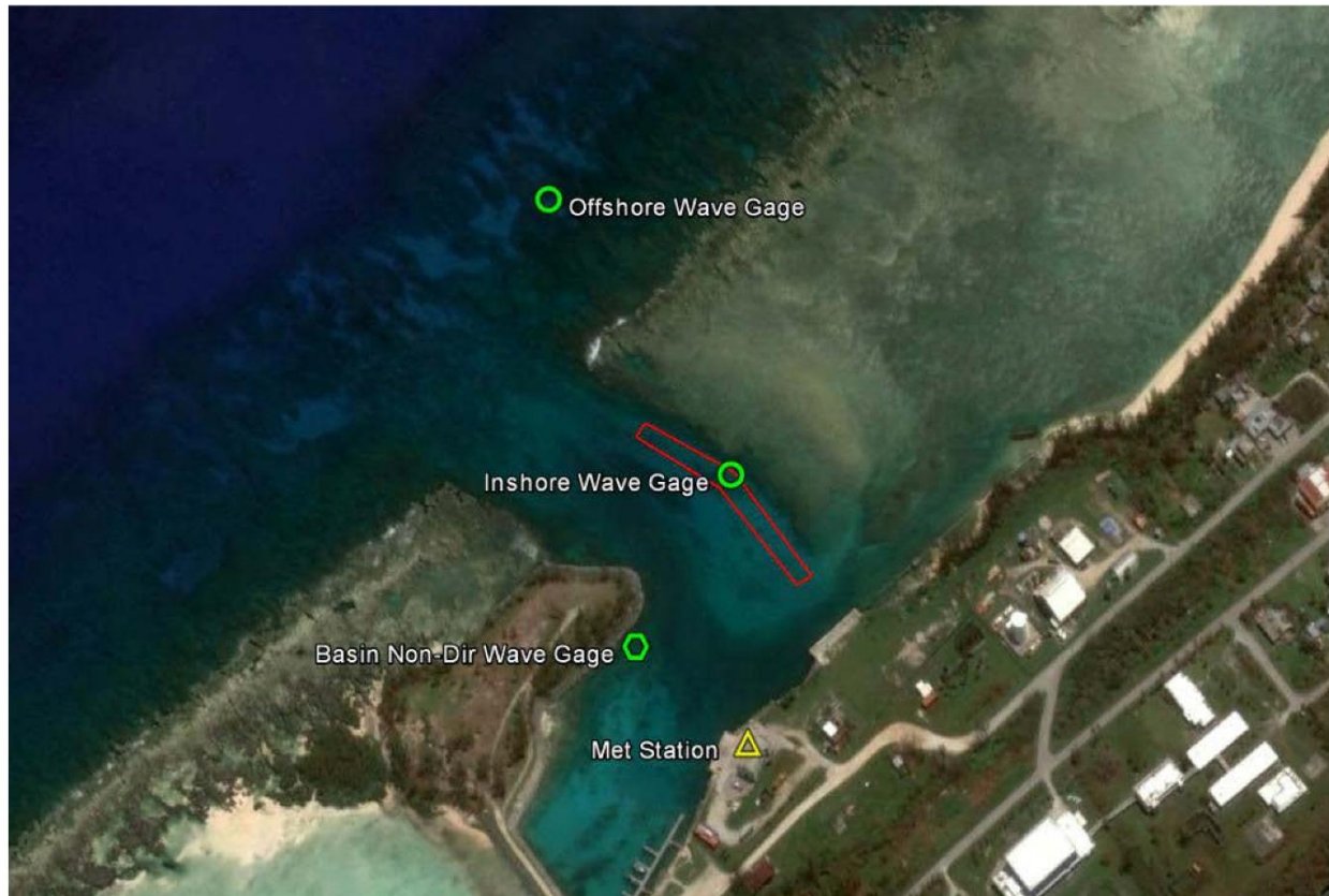
Figure 3. Wave Gage Locations at Rota Island Harbor (Dec. 2, 2016 through Mar. 3, 2017)
