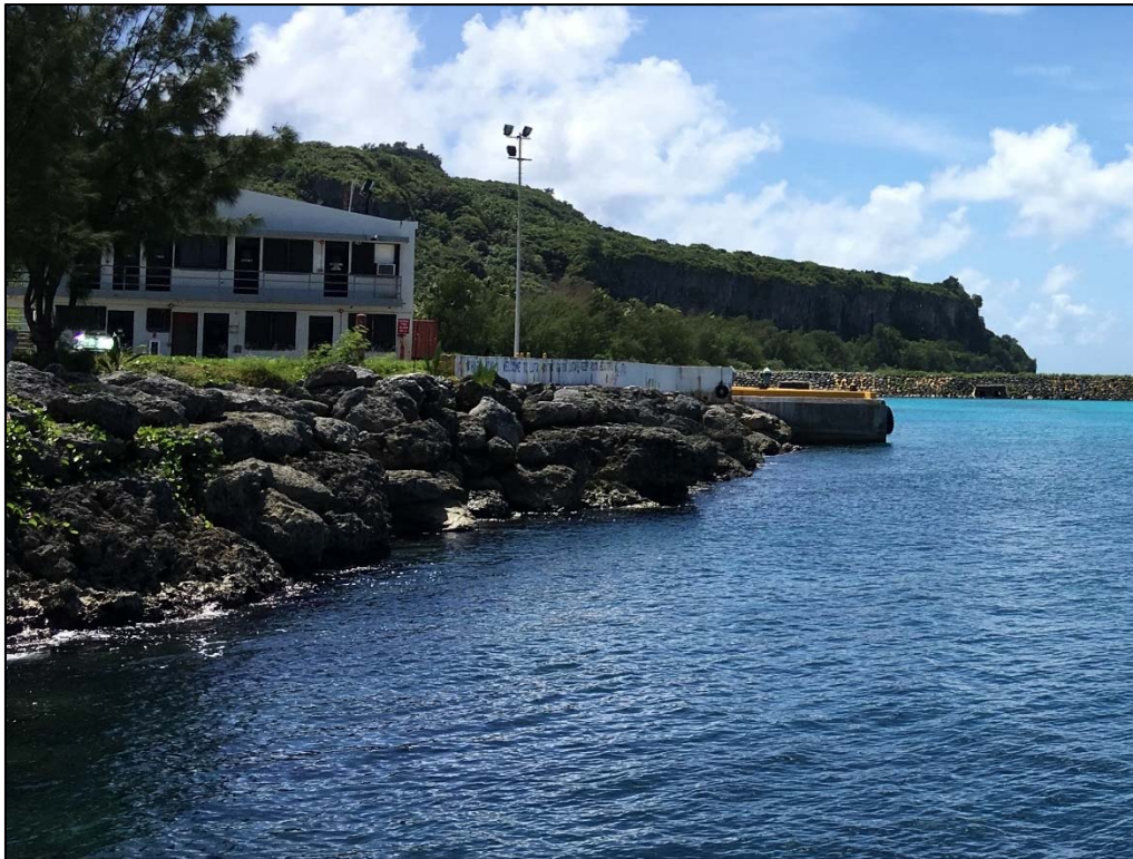
Photo 40. Rock revetment seen from Berth 1 looking south towards Berth 2.
