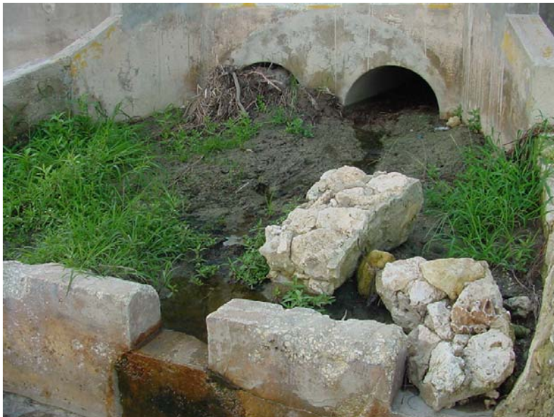
Stormwater runoff outfall point.
