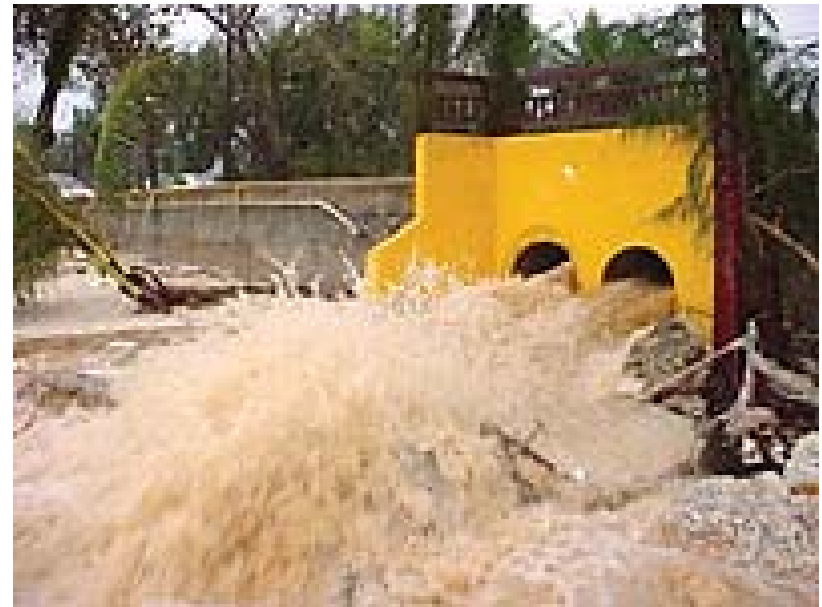
Stormwater runoff during Typhoon Tingting.
