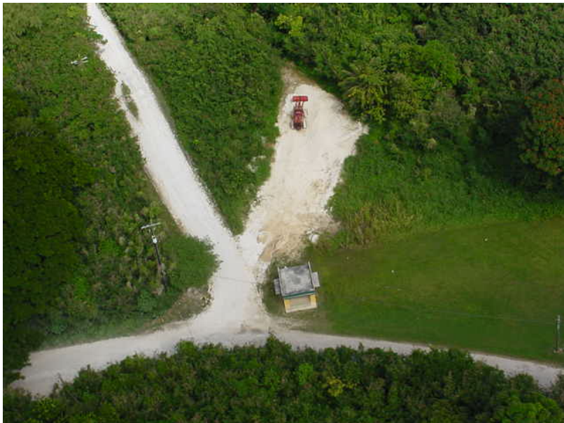
Unpaved roads in West Takpochao watershed.
