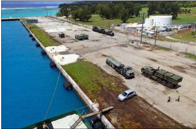
Photo 3-1. North Quay, Berths 1 and 2, North Quay looking west.
