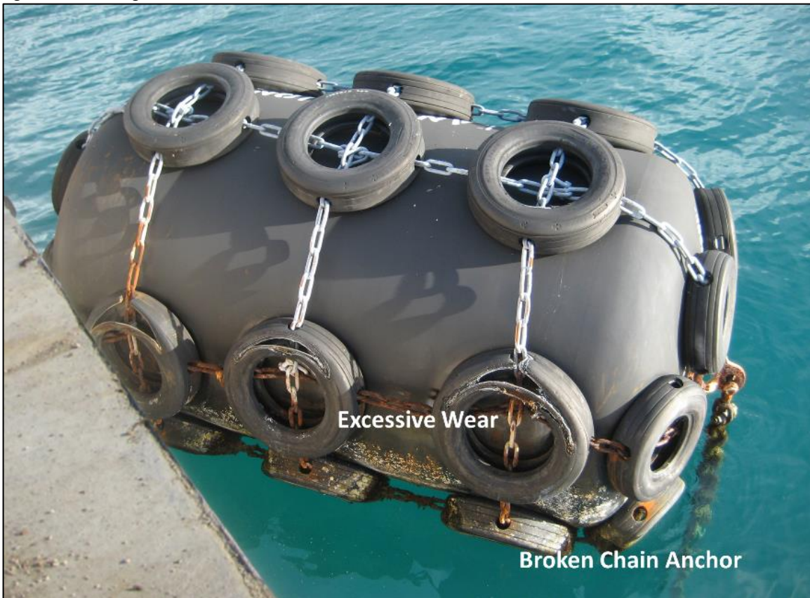
Figure 2-8: Damaged Fender
