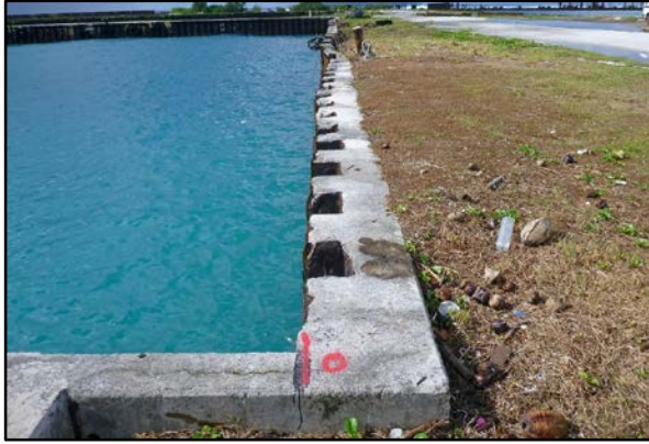
Photo 3-7. East side of the Connecting Pier looking south from North Quay Berth 1.
