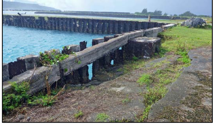
Photo 3-8. Connecting Pier, east side, looking southeast towards Center Finger.
