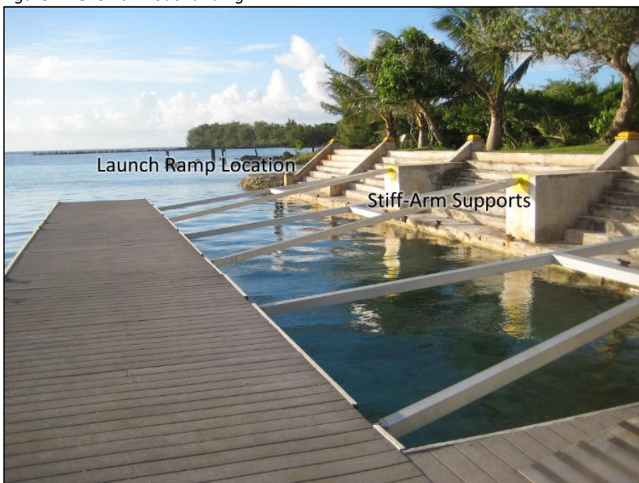
Figure 2-23: Small Boat Landing
