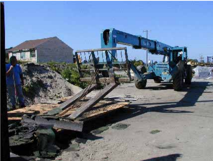
Figure 2.4 Using a “snowplow” to remove asphalt roof shingles. Finding fast, economical tools and methods for Deconstruction is a key step to making it standard practice.
