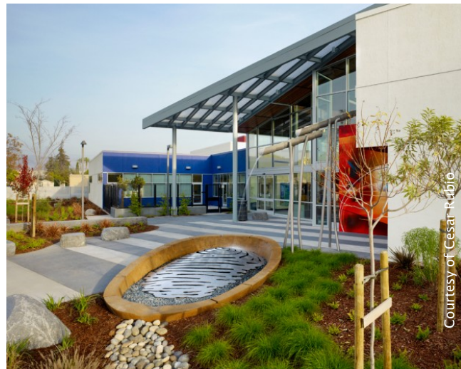
Exhibit 17. Roosevelt Community Center, San Jose, California. The community center incorporates green infrastructure throughout the site, including two installations by artist Jackie Brookner that create a lively public space as well as capture and filter stormwater. Developing the center involved cleaning up and repurposing a former brownfield, which has helped catalyze revitalization of the neighborhood.
