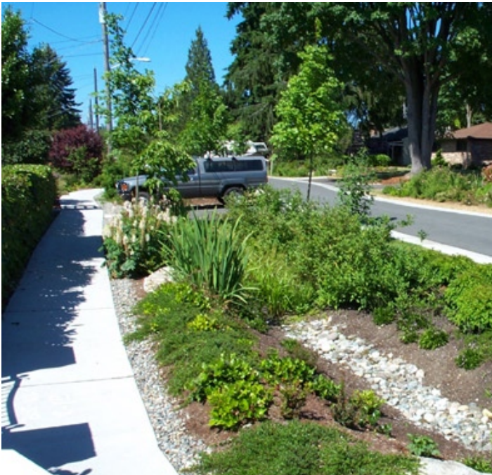
This picture illustrates site level green infrastructure practices such as landscaped swales to capture runoff.
