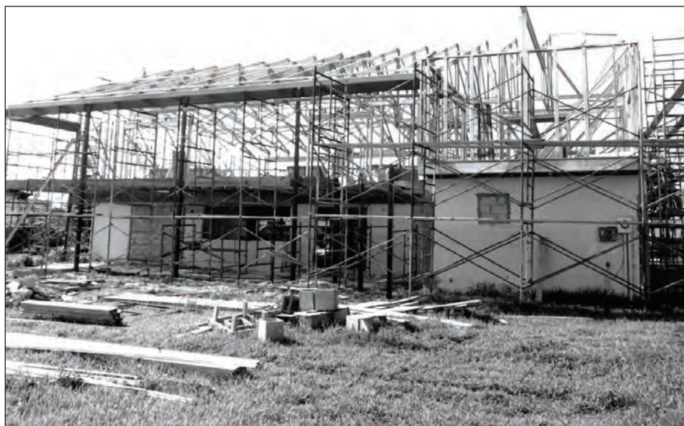
Figure 3-12. The owner of this flood-prone home in south Florida decided to build a new wood-framed second story on top of the masonry first story. The new second story is well above the BFE.
