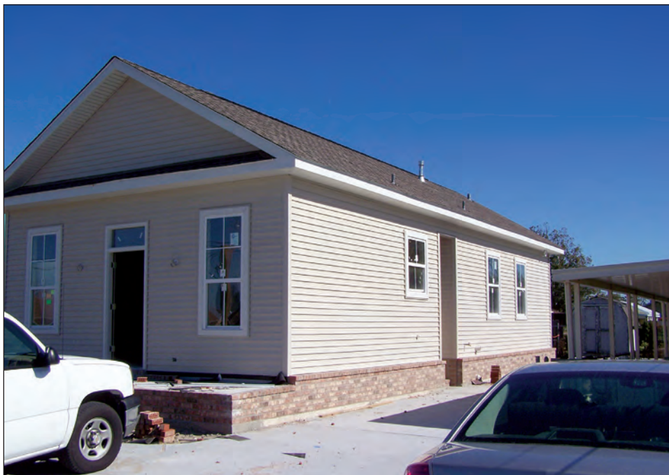
Figure 6-9. Typical mitigation reconstruction project.
