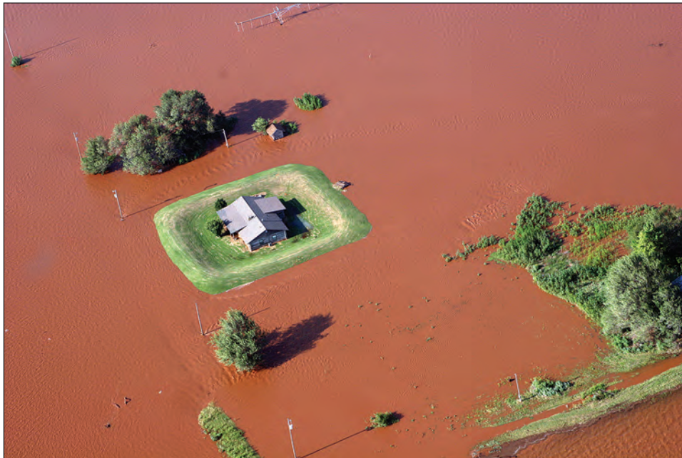
Figure 3-18. A home protected by a levee.
