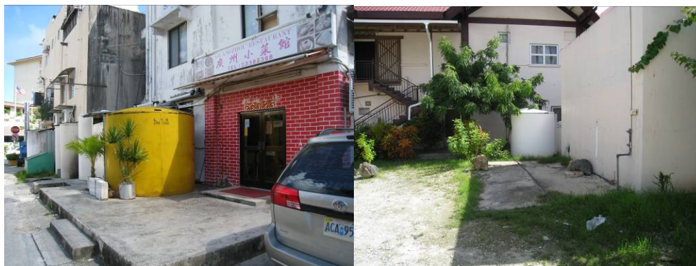
Figure S4.1. Examples of rainwater harvesting for backup potable and other uses on Saipan
