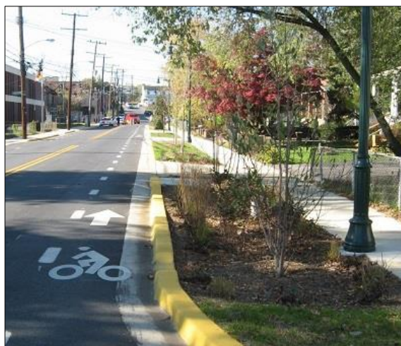
Figure 22: This street in Edmonston, Maryland, incorporates green infrastructure elements, including pervious paving in the bike lane, while making the street pleasant and safe for all users.
