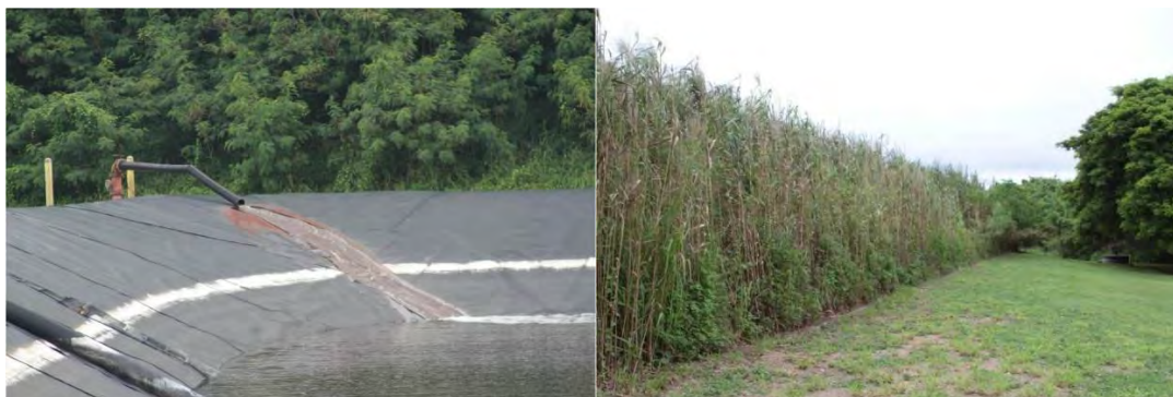
Figure 6. Lined leachate pond (left) and wetland leachate treatment system (right)
