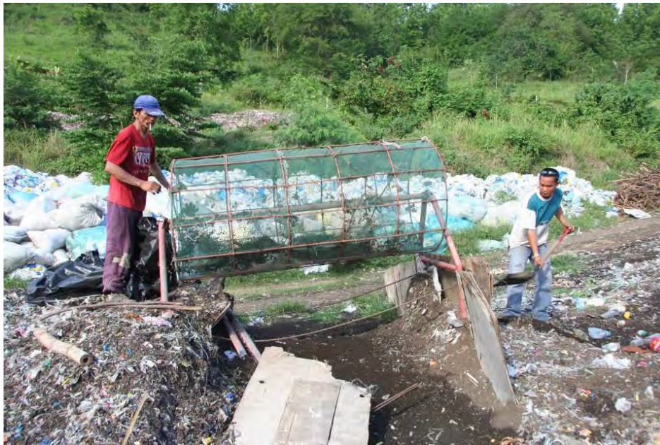
Figure 27. Equipment built for screening compost
