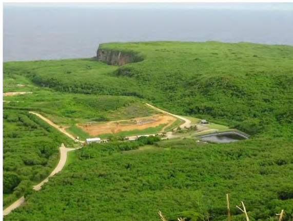
Figure 5. Aerial view of the Marpi Landfill in Saipan, CNMI
