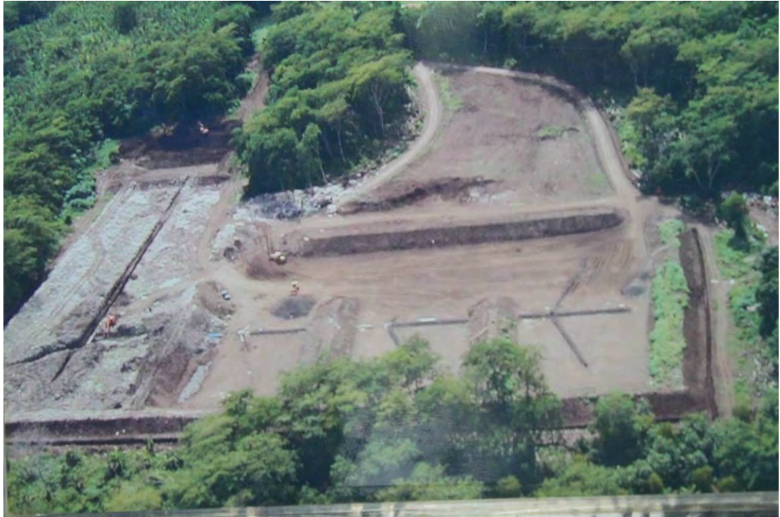
Figure 16. Historic image showing the construction of the Tafaigata Fukuoka-style Landfill
