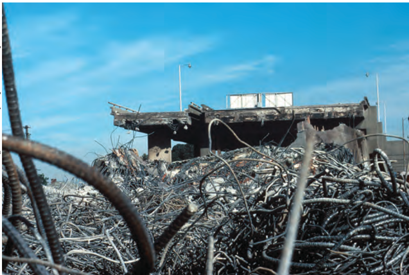
Figure 1.2. Reinforcement bars lie at the base of the Cypress Viaduct of Interstate 880, Oakland, California, October 17, 1989.
