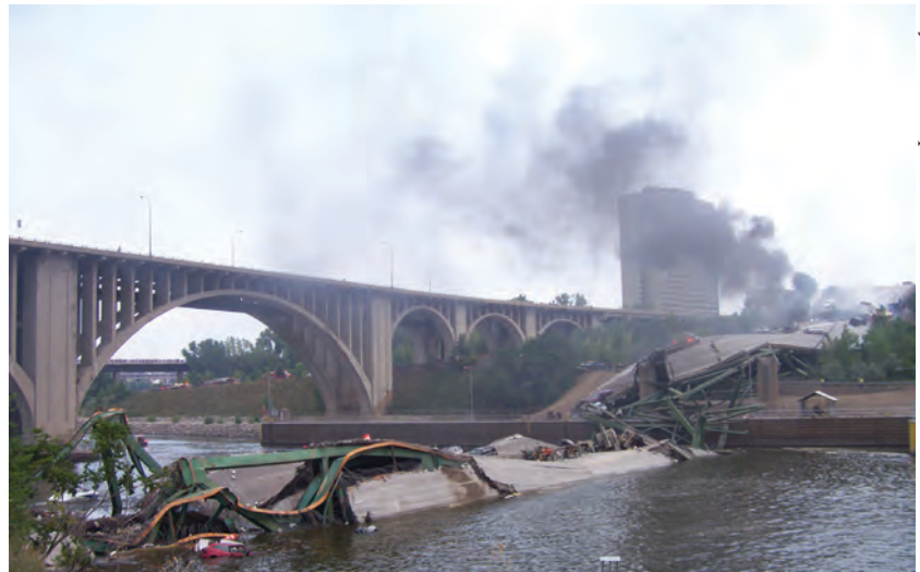
Figure 3.4. The Interstate 35W bridge in Minneapolis, shortly after its 2007 collapse
