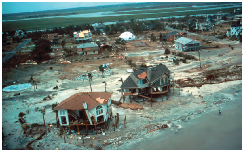
Figure 3.3. Damage by Hugo to South Carolina's Isle of Palms
