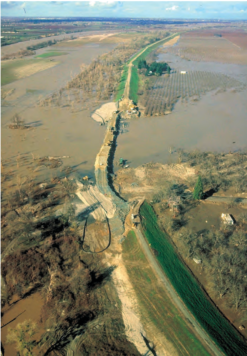
Figure 4.1. Aerial view of a broken levee and the resultant flooding on the Sacramento River in the Sacramento River delta
