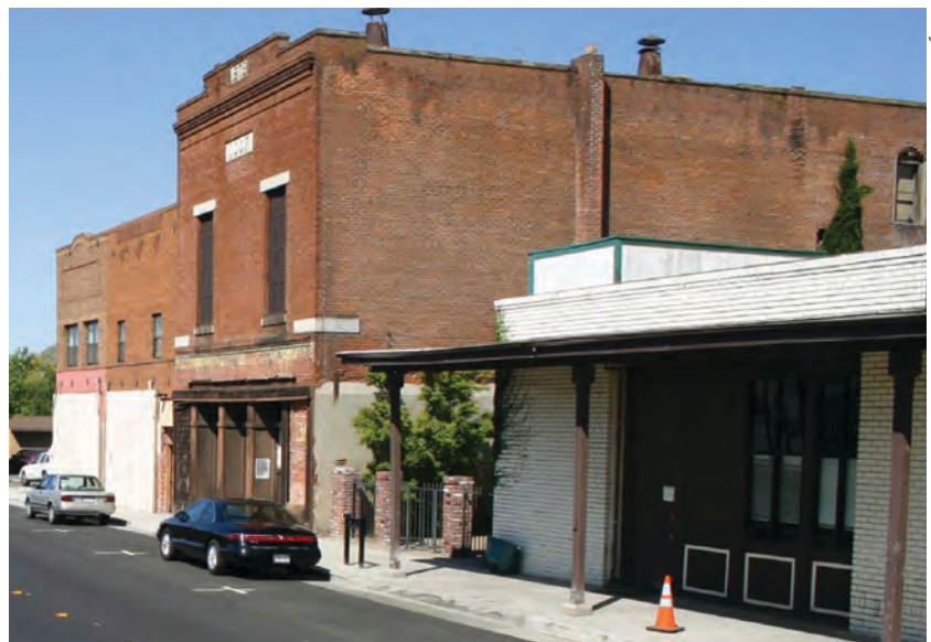
Figure 7.7. Downtown area unreinforced masonry buildings
