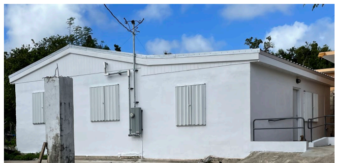
Figure 2. Example of a building updated with building envelope retrofits.
