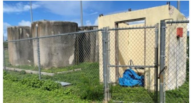
**Figure 5. Examples of critical building system damage: water pump enclosure damage and water reservoir in need of maintenance.**
