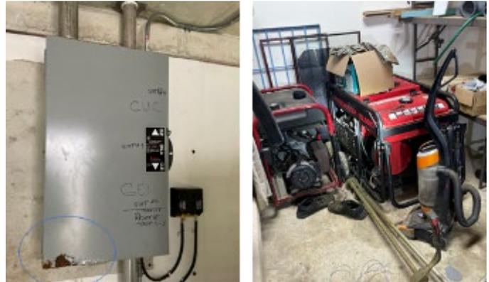
**Figure 3. Examples of electrical system damage: corrosion on electrical panel (left) and non-functioning generators (right) see recommendation 3.**
