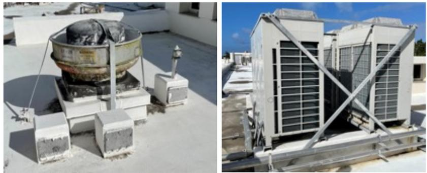
**Figure 2. Examples of correctly braced HVAC rooftop units and equipment with little or no damage.**
