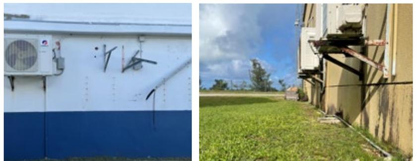
**Figure 1. Examples of HVAC damage: blown off mini-split system (left) and corroded wall bracket (right).**
